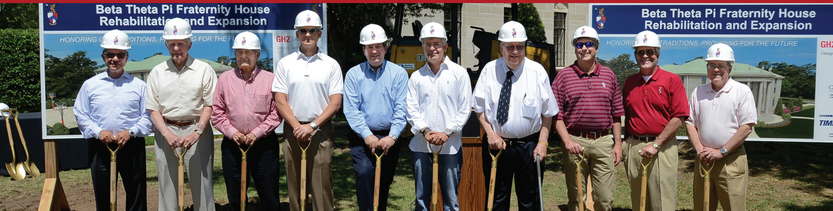
Campaign leadership was on hand to begin the work for the chapter's renovation. Your support is needed during this exciting time in the chapter's history.
